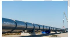
system that uses evacuated tubes to move multipassenger vehicles at speeds up to 700 mph. Several companies are currently developing prototypes, and planning has been started to deploy the systems in routes in several key markets within the U.S.
